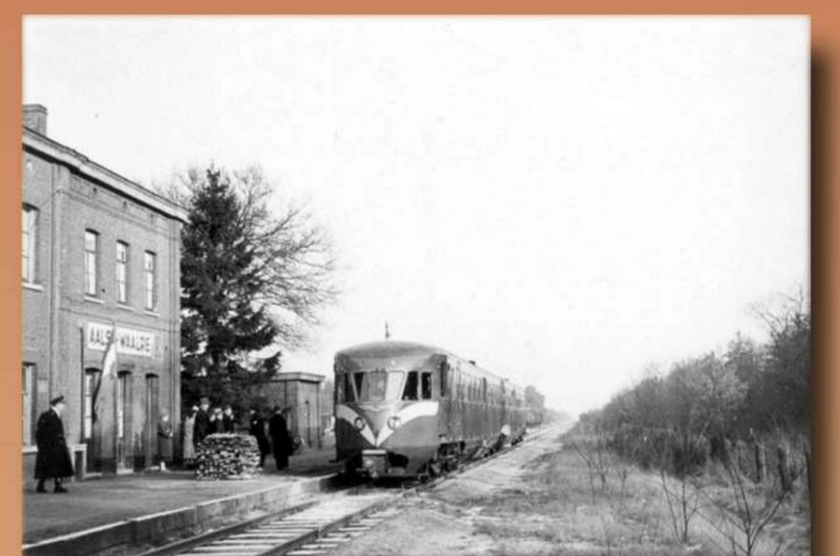
Station Aalst Waalre
